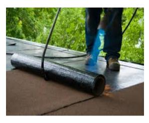
• **Description**: Flat roofs are often used in commercial buildings and require specific materials (like TPO, EPDM, or modified bitumen) that can withstand pooling water. They typically have a slight pitch for drainage.
