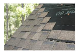
**Description**: This process involves laying down individual shingles, typically made of asphalt, wood, or metal, in overlapping rows to create a waterproof barrier on sloped roofs. Proper installation is crucial
