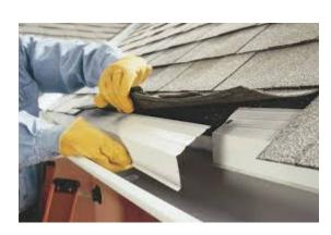
• Description: A drip edge is a metal flashing installed at the roof's edge to guide water away from the fascia and prevent
